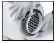
Fit foam collar seal around inlet spigot (supplied with unit).
