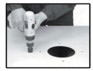
Cut hole for oil return tube (if required).
